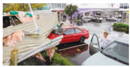
Iron from a roof on top of cars parked at the Albany Mega Centre. Photo: Brett Phibbs.
